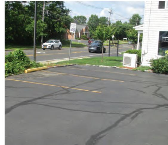
Parking spaces located in the south section of the parking lot can be replaced with pervious pavement to capture and infiltrate stormwater. Downspouts at Annie's Deli can be disconnected and directed into downspout planter boxes to capture and filter rooftop runoff. A preliminary soil assessment suggests that more soil testing would be required before determining the soil's suitability for green infrastructure.
