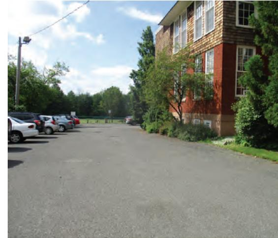
Bioretention systems can be installed southeast of the southernmost building and southeast of the tennis court to capture, treat, and infiltrate rooftop, tennis court, and parking lot runoff. Parking spaces located to the west of the northernmost building can be replaced with pervious pavement to capture and infiltrate stormwater. A preliminary soil assessment suggests that more soil testing would be required before determining the soil's suitability for green infrastructure.
