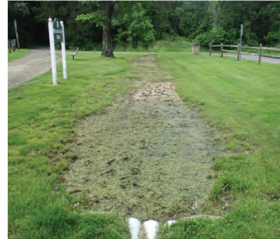
Connected bioretention systems can be installed on the eastern edge of the parking lot to capture, treat, and infiltrate runoff. The systems can be linked by pipes (already installed) shown in the above image. Pervious pavement can be installed in the parking spaces on the southern edge of the parking lot to filter and infiltrate pavement runoff. A preliminary soil assessment suggests that more soil testing would be required before determining the soil's suitability for green infrastructure.
