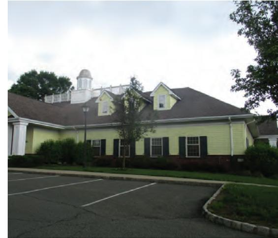
Bioretention systems can be installed to capture, treat, and infiltrate rooftop runoff on the north and south of the building. Pervious pavement can be installed in the southeast corner of the parking lot to capture and infiltrate stormwater. A preliminary soil assessment suggests that the soils have suitable drainage characteristics for green infrastructure.
